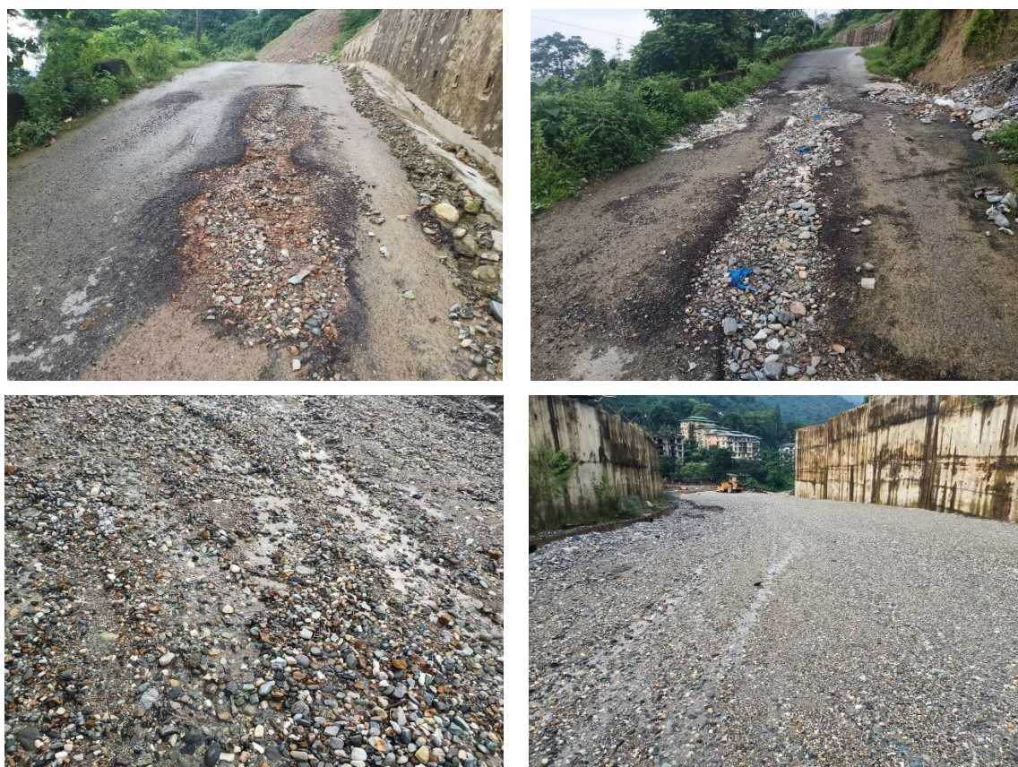
Figure 4. Post and pre-condition of pavement surface and base layers due to poor quality control measures
