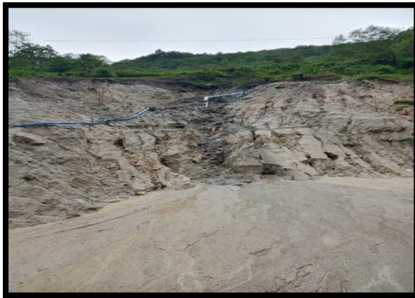
Figure 3. (a) Fan-Shaped colluvium material deposit at the base of the slope; (b) Water diversion using wooden catch basin
