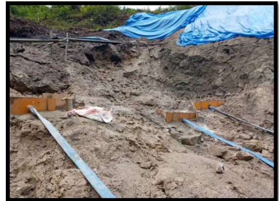
Figure 3. (a) Fan-Shaped colluvium material deposit at the base of the slope; (b) Water diversion using wooden catch basin
